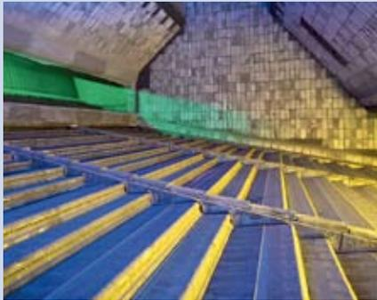
High-tech combustion chambers using grate technology guarantee an optimum process with low emissions and high residue quality.
